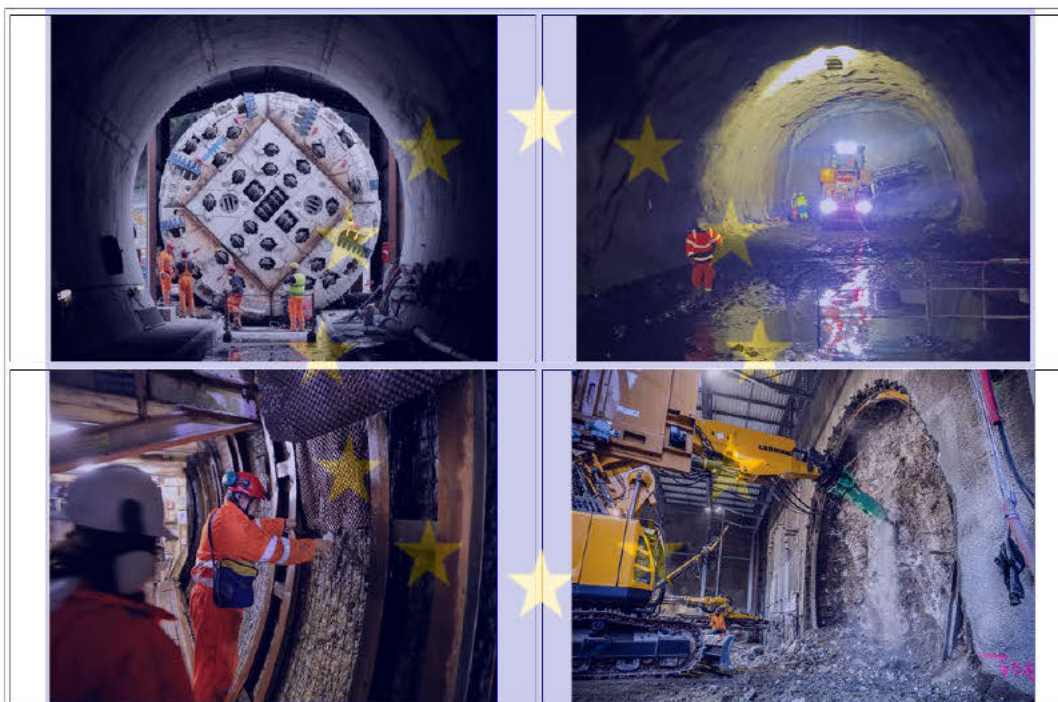
Works for the construction of the base tunnel of the Mont Cenis
