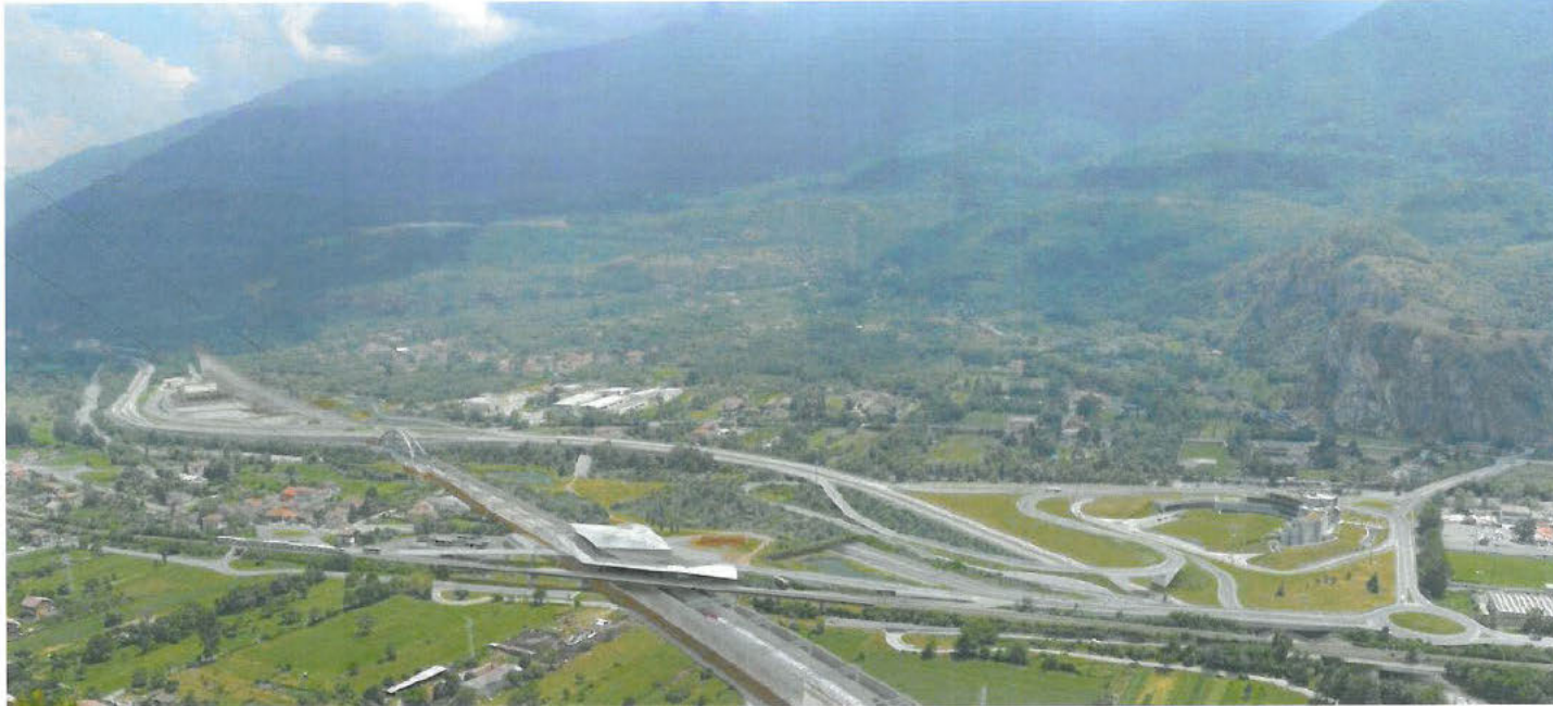
Lay out of the Susa Plain after the completion of the works
