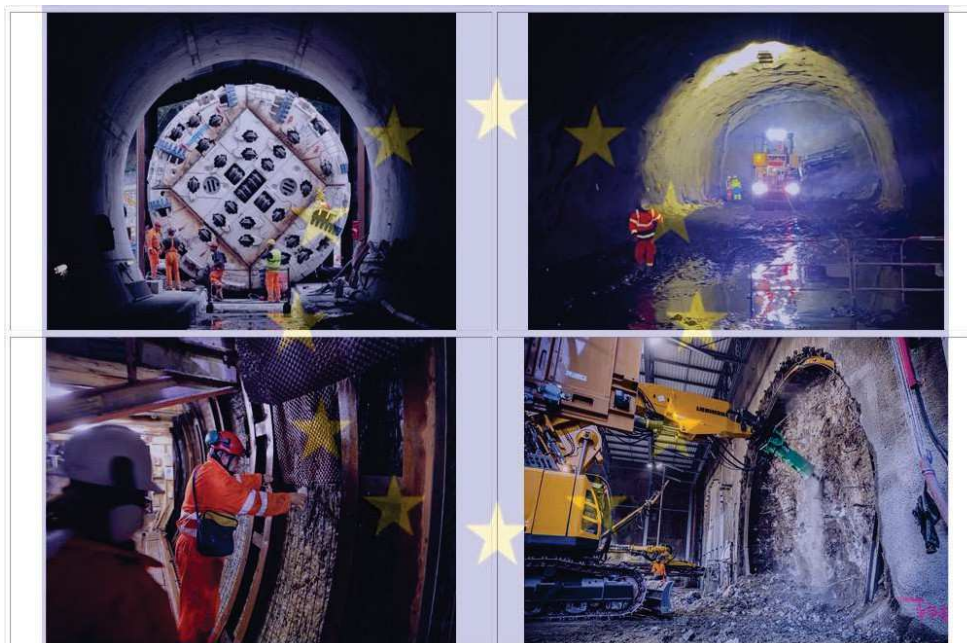
Works for the construction of the Mont Cenis base tunnel
